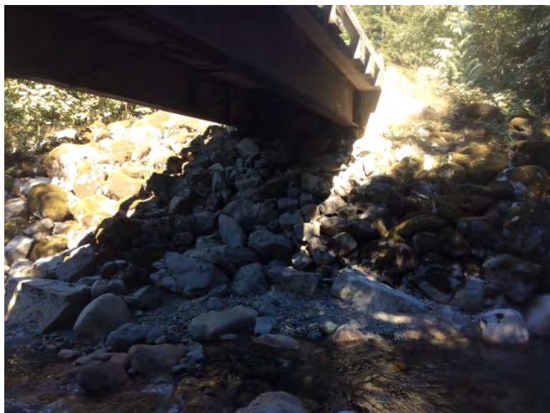
Right Bank Abutment when facing downstream
