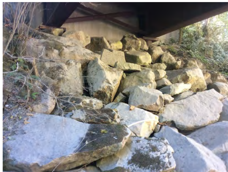
Left Bank Abutment when facing downstream
