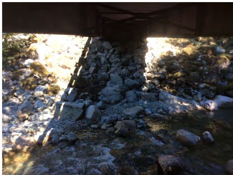
Right Bank Abutment when facing downstream
